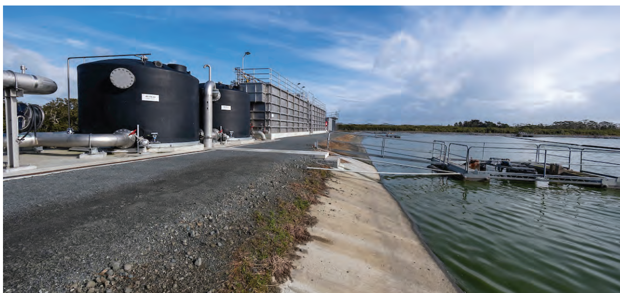
Figure 14 - Te Awaroa (Helensville) WWTP June 2023
