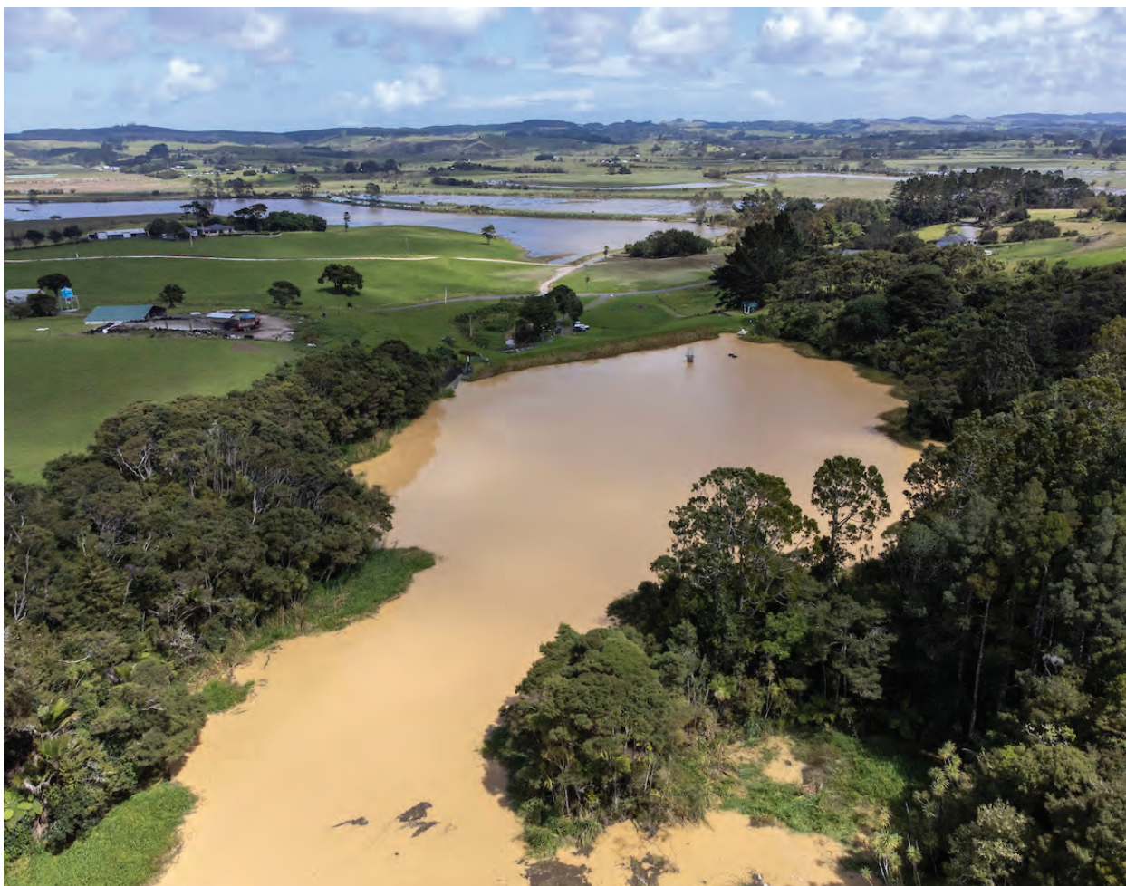
Figure 4 - Mangakura Dam Feb 2023
