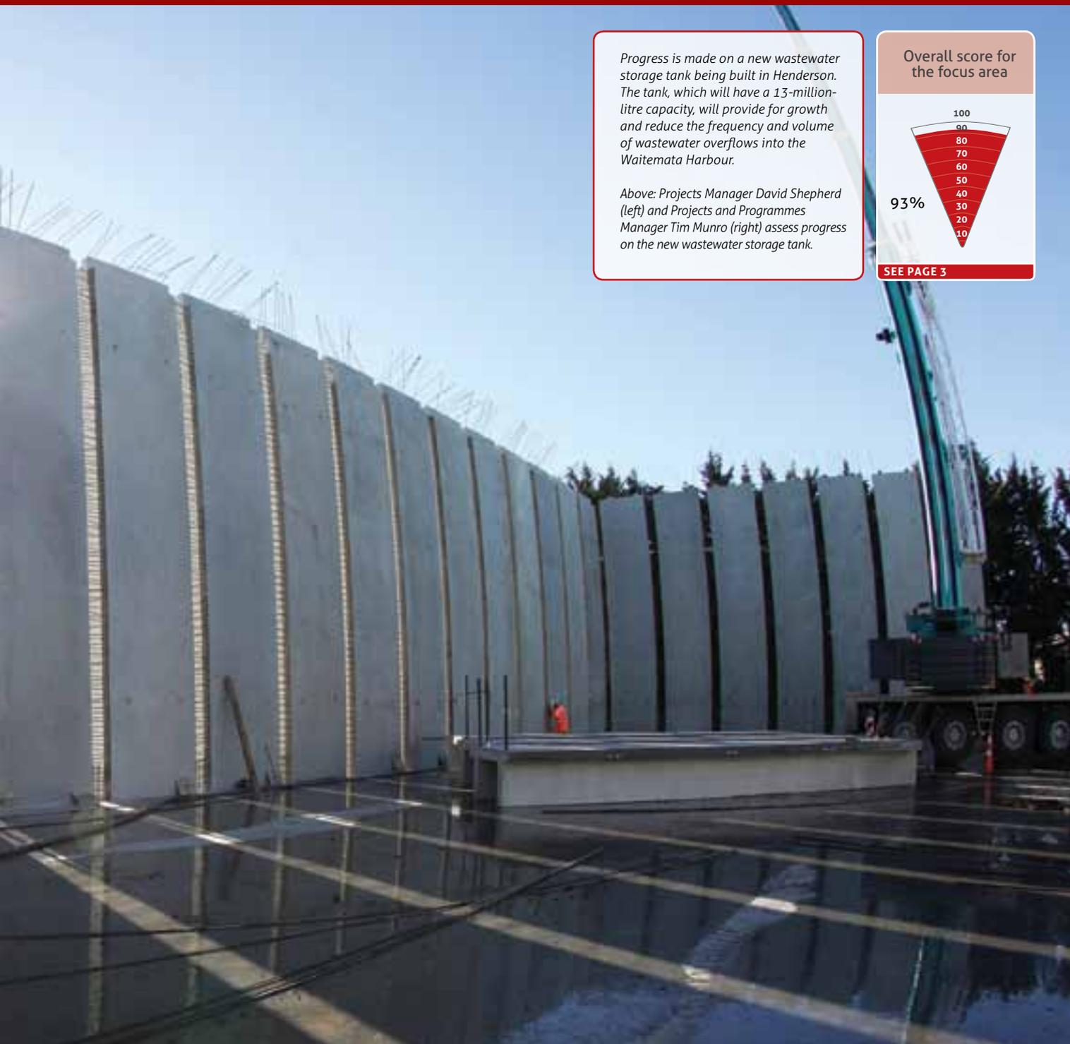
*Progress is made on a new wastewater storage tank being built in Henderson. The tank, which will have a 13-million-litre capacity, will provide for growth and reduce the frequency and volume of wastewater overflows into the Waitemata Harbour.*
