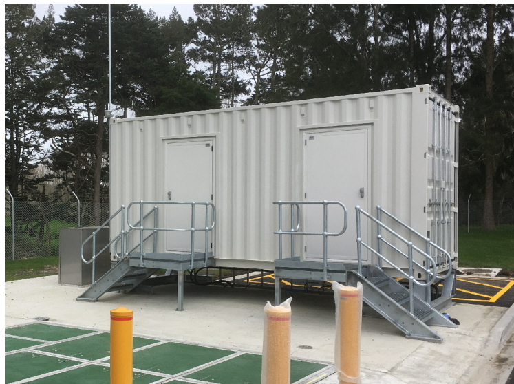
TYPICAL CONTAINER INSTALLATION FOR A PUMP STATION
