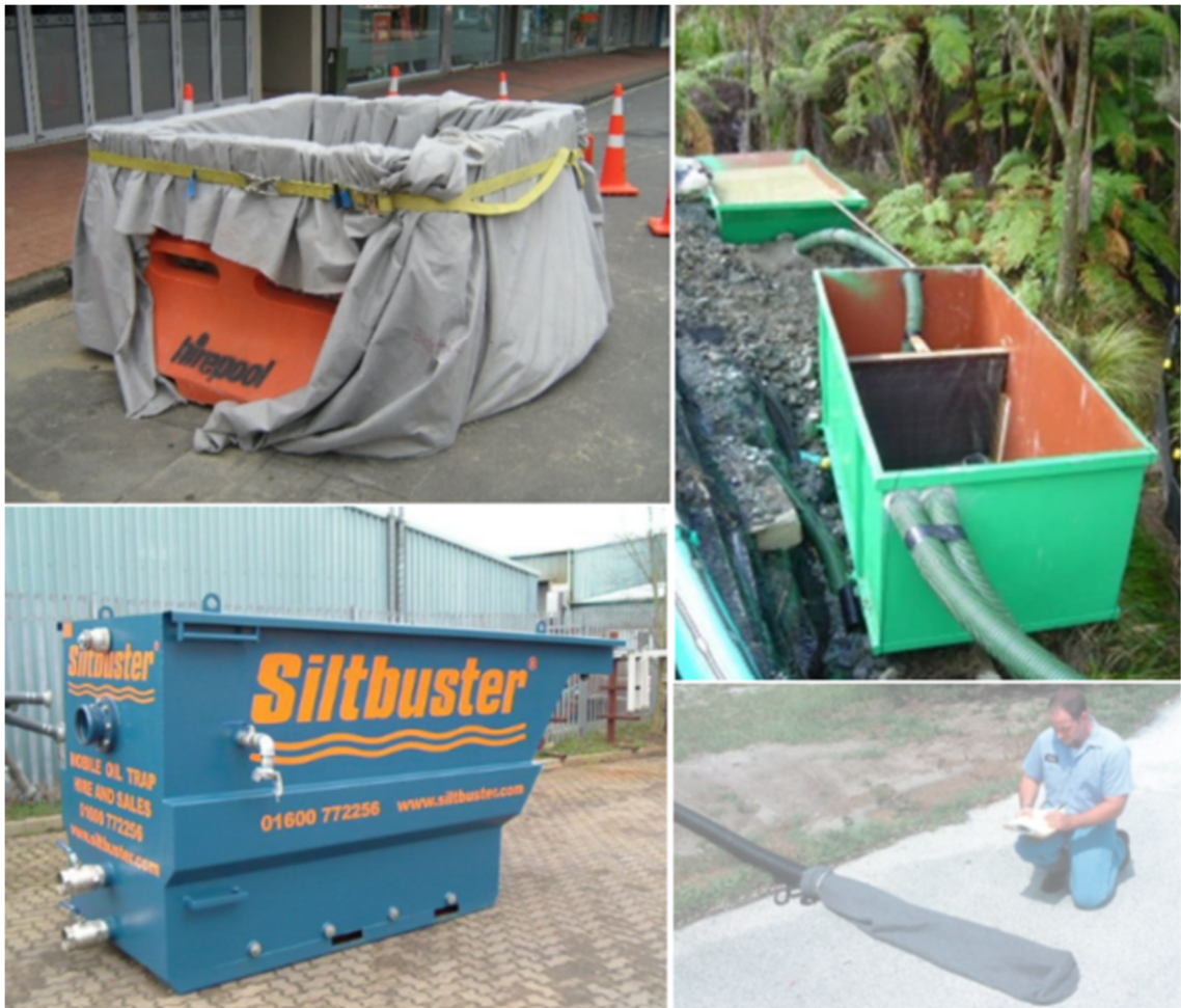
Figure 7. Example dewatering devices, clockwise from top left: turkeys nest, baffled skip bins, small dewatering bag, lamella clarifier.
