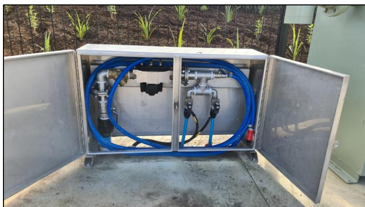
Figure 7: Example water supply cabinet.
