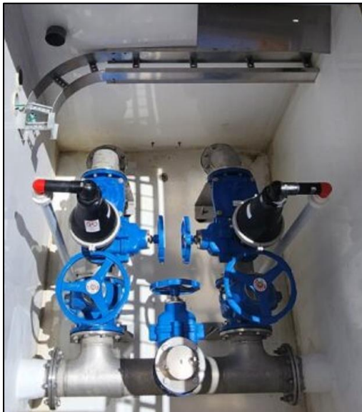
Figure 4: Example of valve arrangement on discharge side of wet well.
