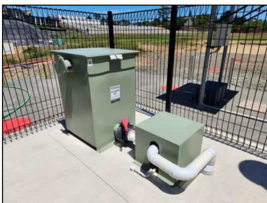
Figure 6: Example of an odour control system installed and treating wet well odour.
