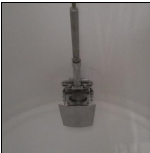
Figure 5: Example of knife gate valve at the inlet to the wet well including extension spindle.
