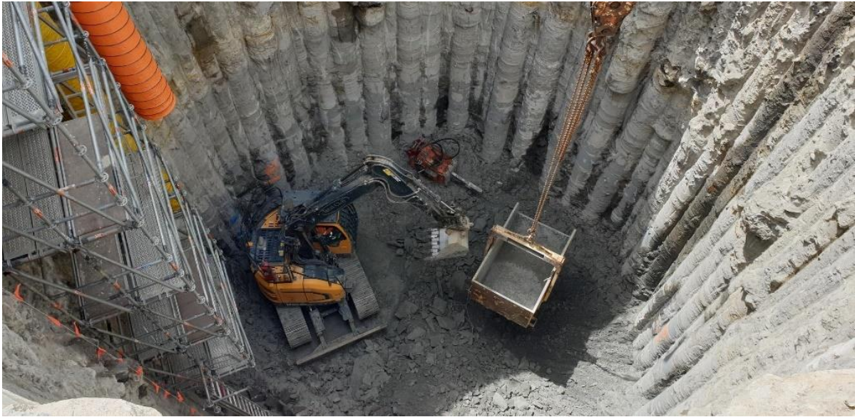
Figure 3-12. Example of construction of a shaft for a TBM (Photograph: Rachael Clark, 20 th October, 2022)
