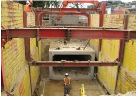
Figure 22. Example of the double slide rail trench support system (Source: https://www.shorenz.co.nz/Double_Rail_Systems.php )
