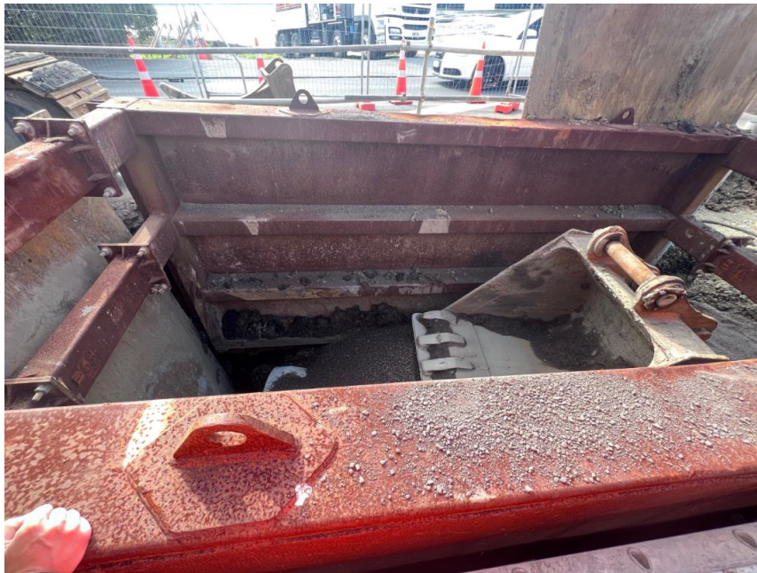
Figure 4-10. Example of open trenching using trench shields (Photograph: Tingran Duan, 2 September 2022)
