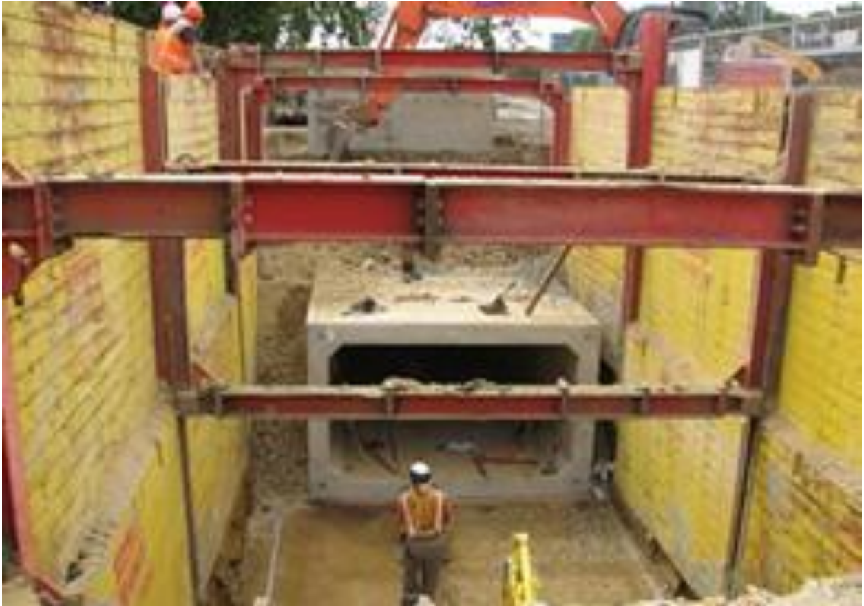
Figure 4-8. Example of the double slide rail trench support system (Source: https://www.shorenz.co.nz/Double_Rail_Systems.php )
