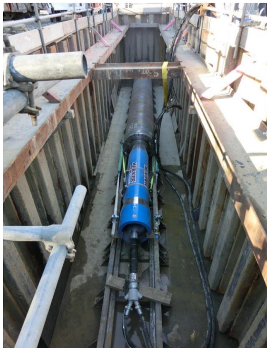
Figure 4-11. Photograph of indicative pipe hammering set up (Source: Brian Perry Civil)
