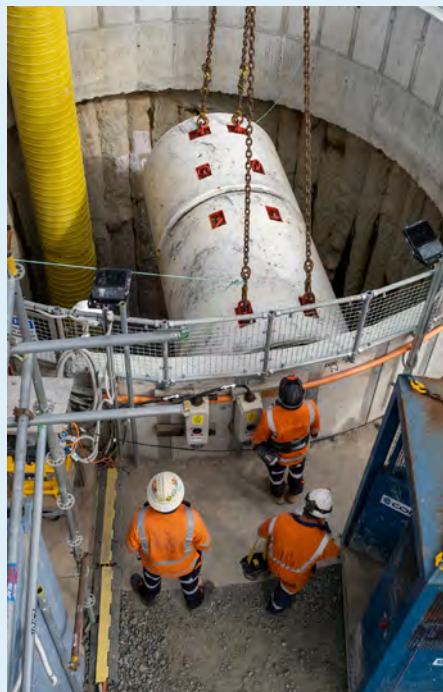
The mTBM being lowered into a shaft on the Central Interceptor project
