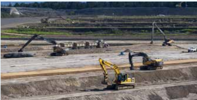
Biosolids operation on Te Motu a Hiaroa (Puketutu Island).
