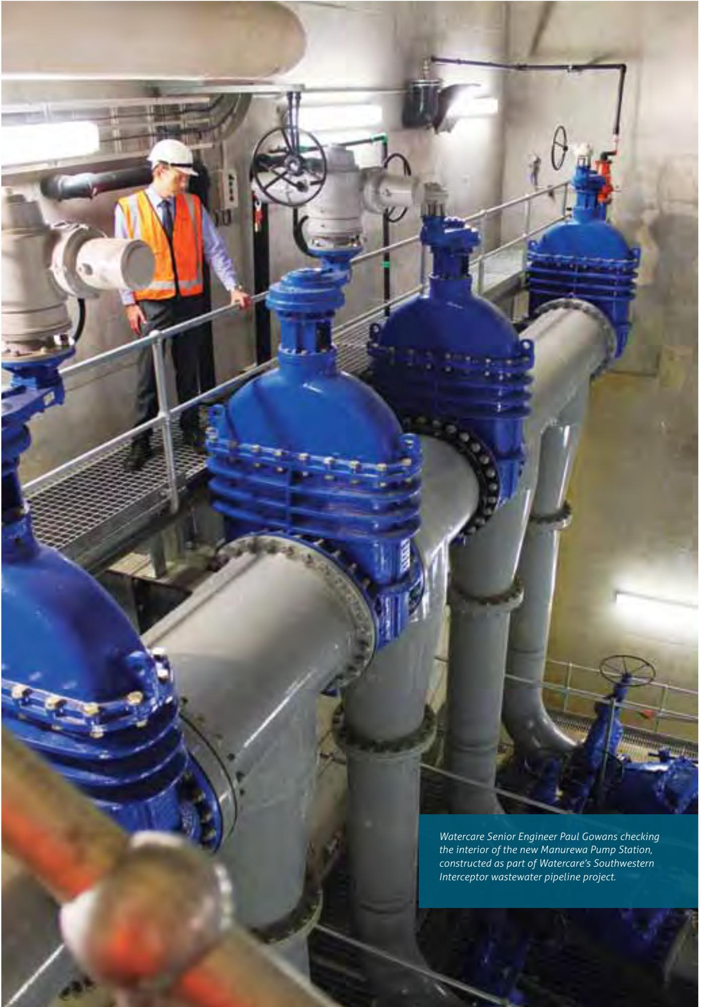
*Watercare Senior Engineer Paul Gowans checking the interior of the new Manurewa Pump Station, constructed as part of Watercare's Southwestern Interceptor wastewater pipeline project.*
