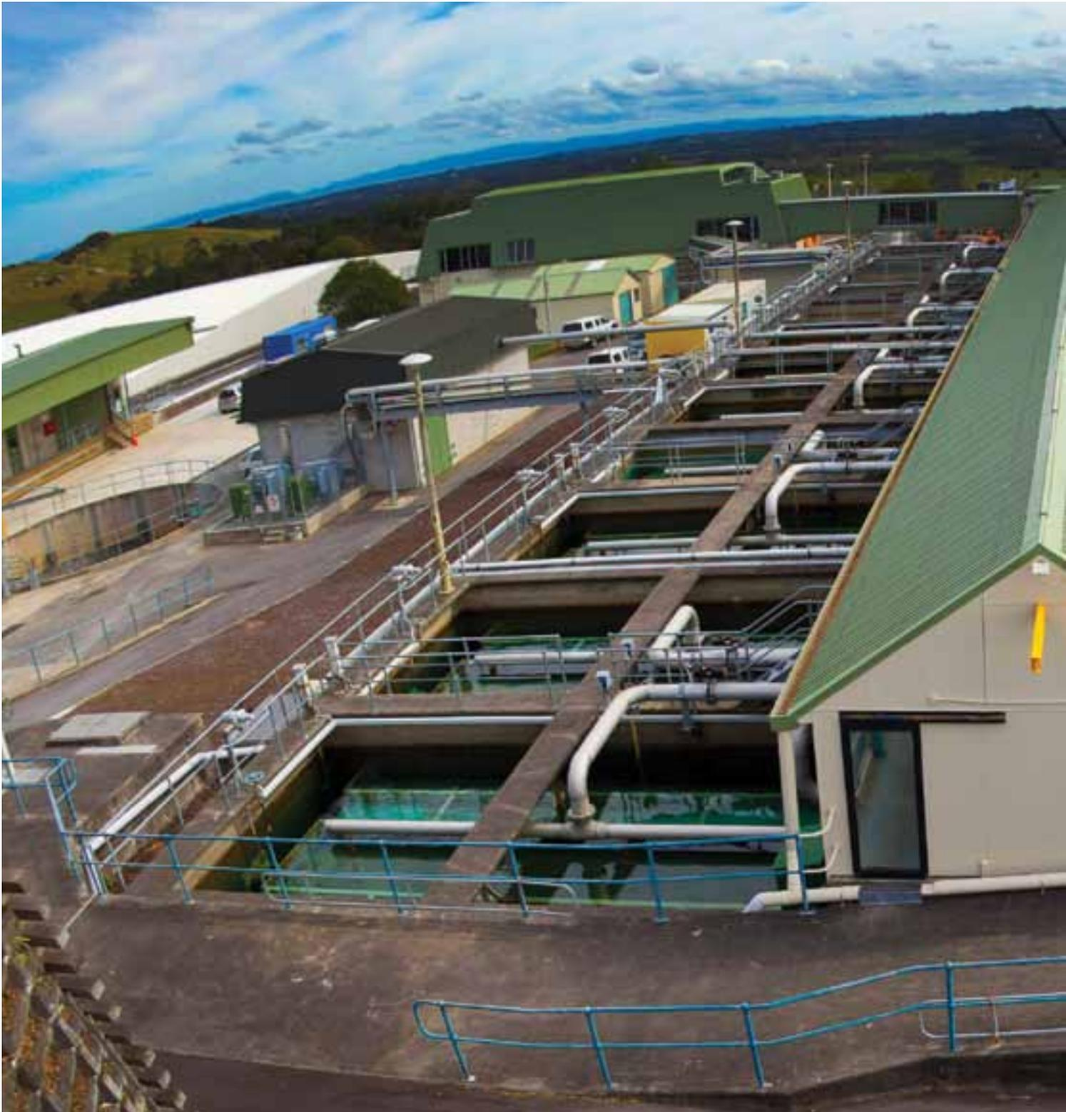
*Sedimentation beds at Ardmore Water Treatment Plant, where settlement of suspended solids takes place as part of the water treatment process.*
