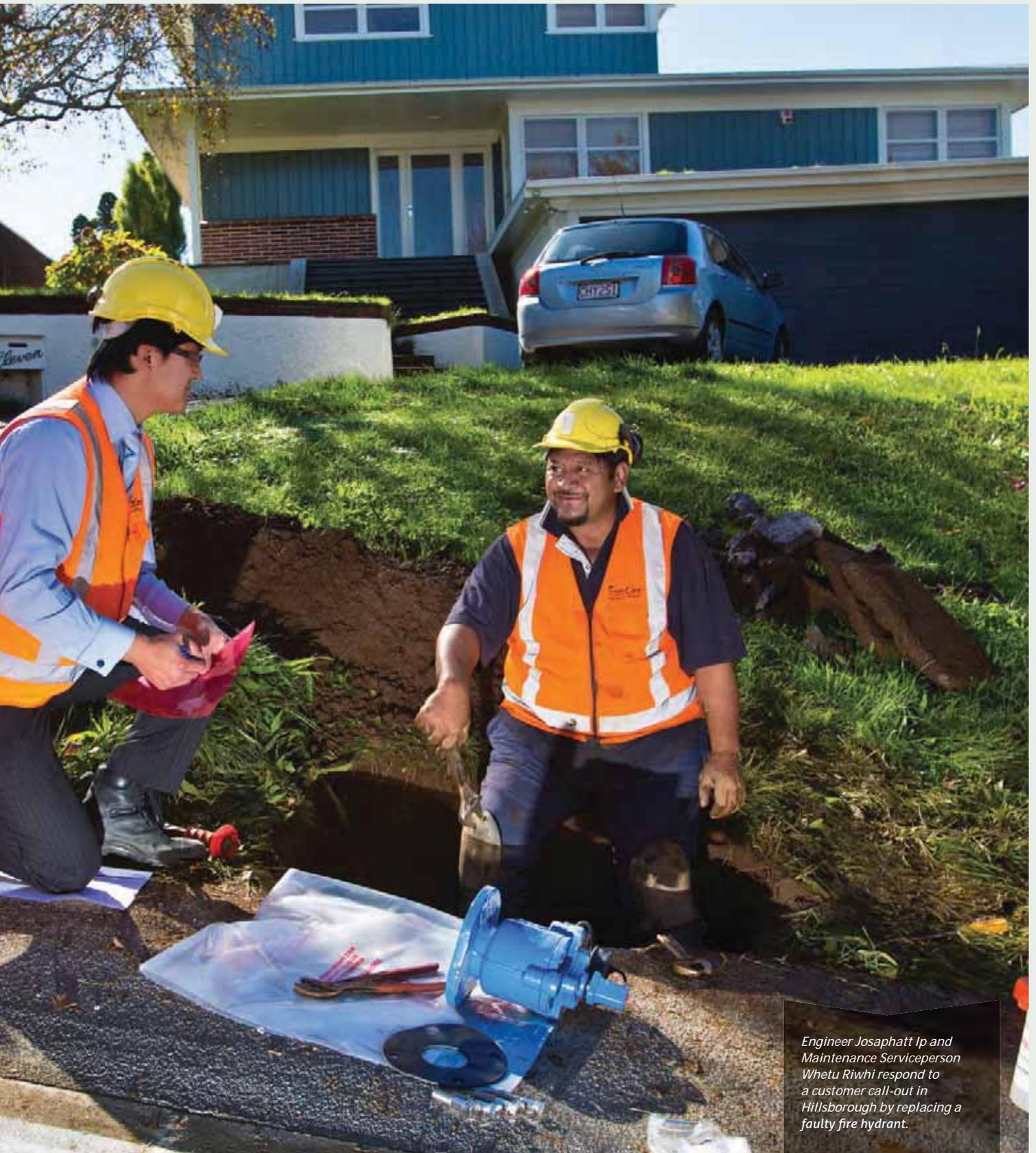
*Engineer Josaphatt Ip and Maintenance Serviceperson Whetu Riwahi respond to a customer call-out in Hillsborough by replacing a faulty fire hydrant.*
