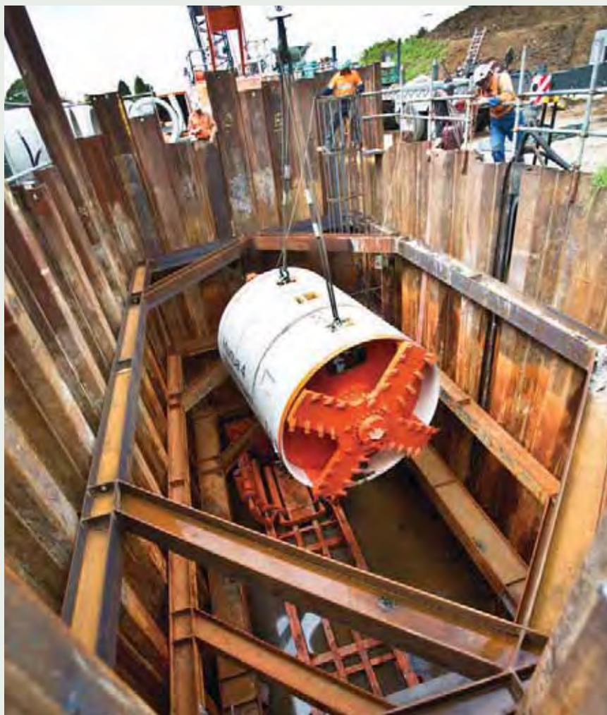
*A section of a tunnel boring machine is lowered into a shaft as part of the Hunua 4 watermain project. The machine was used to pass underneath State Highway 1 in Flat Bush as it was not feasible to complete this section using an open trench.*
