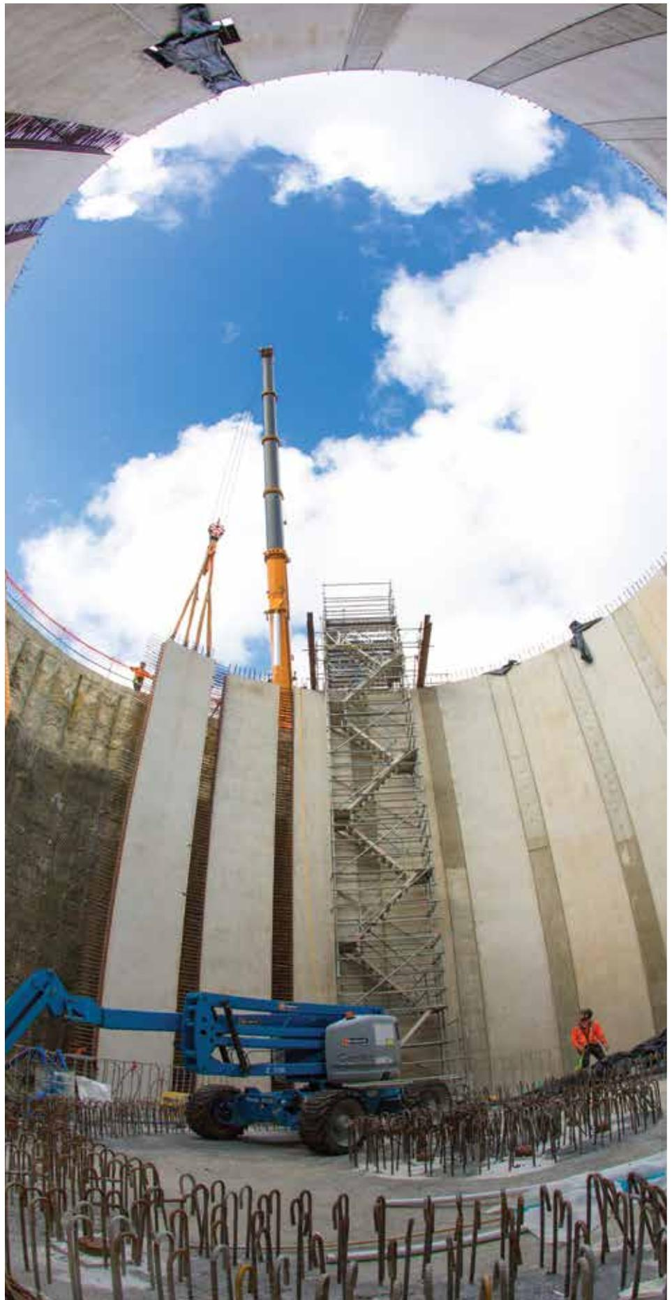
*Watercare is constructing an underground storage tank in Madills Farm Reserve as part of a wider project to upgrade the wastewater network that services the east Auckland suburb of Kohimarama. The tank will improve beach water quality by reducing the frequency of wet weather overflows into the creek at Madills Farm Reserve.*
