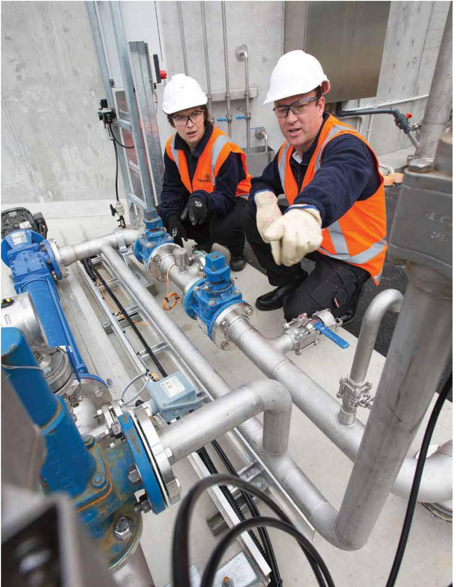
*Water Supply Manager Nolwenn Lagadec discusses the new thickened sludge pump arrangement at Waikato Water Treatment Plant with Operations Controller Stuart Urquhart.*
