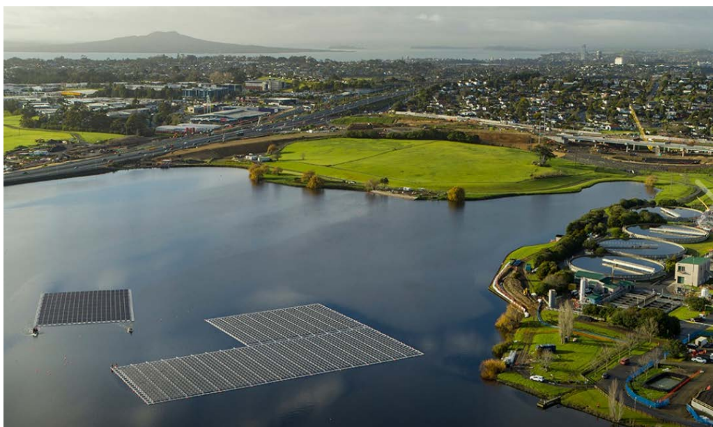
The final piece of the floating solar array at our Rosedale Wastewater Treatment Plant being towed into place
