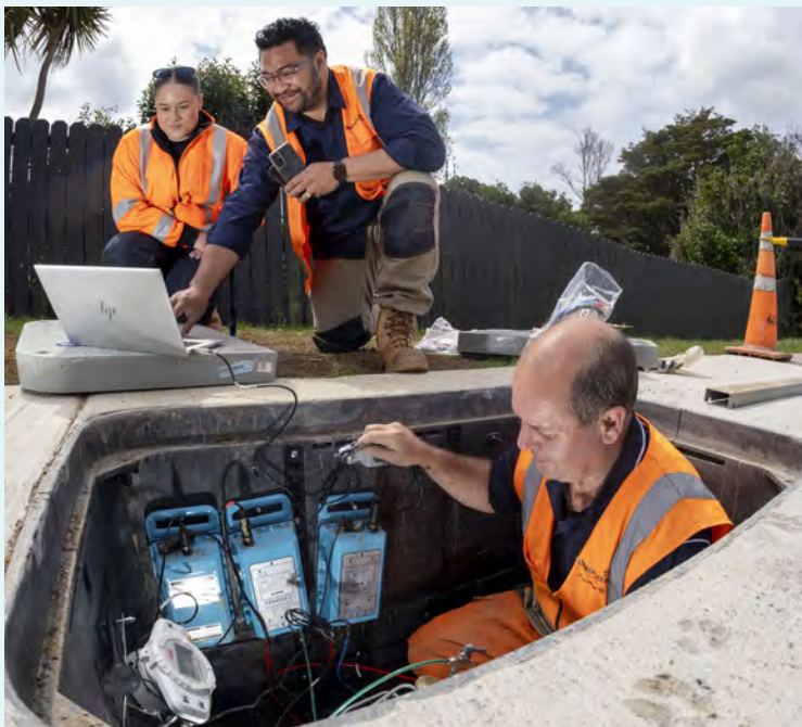
Watercare graduate engineer Tina McIntosh, Watercare smart network engineer Finau Pole and CityCare planned team leader Young Prole install a pressure controller in a pressure-reducing valve chamber in Cockle Bay.
