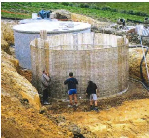
Figure 6 – (a) Construction of underground tanks at Owhanake. (b) Aerial view of completed Owhanake wastewater treatment plant in 2002. (Source: Rob Tinholt and Rick Soar (2002) Treating Waiheke's Wastewater )
