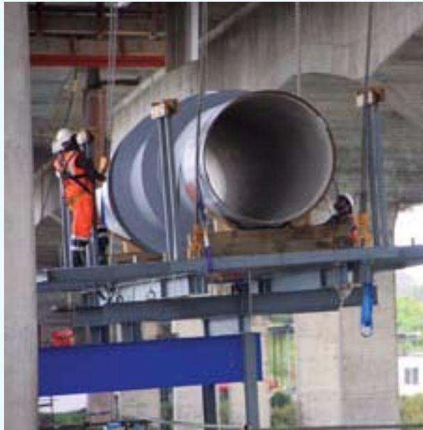
A section of the Hunua No. 4 Watermain is lifted into position under the Manukau Harbour Bridge.
