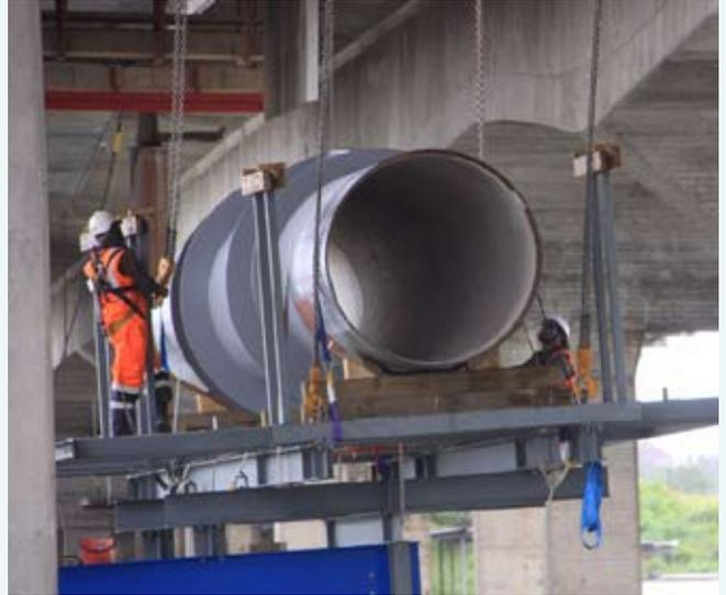
Contractors install an 8.5-metre-long section of watermain on the new Manukau Harbour Bridge.
