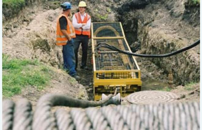
Project Engineer Richard Weaver (right) and a contractor prepare to pull a polyethylene pipe through Hunua No. 1 Watermain using a custom-made winch.
