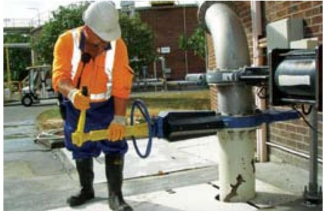
Plant Operator Nigel Prentice opens an isolation valve at the Mangere Wastewater Treatment Plant using a valve-exercising ratchet designed by him and Shift Engineers John Sutherland and Allan Julian. Their tool makes the opening and closing of these valves easy, whereas it used to take time and muscle power. The innovation was recognised with a Continuous Improvement Award.
