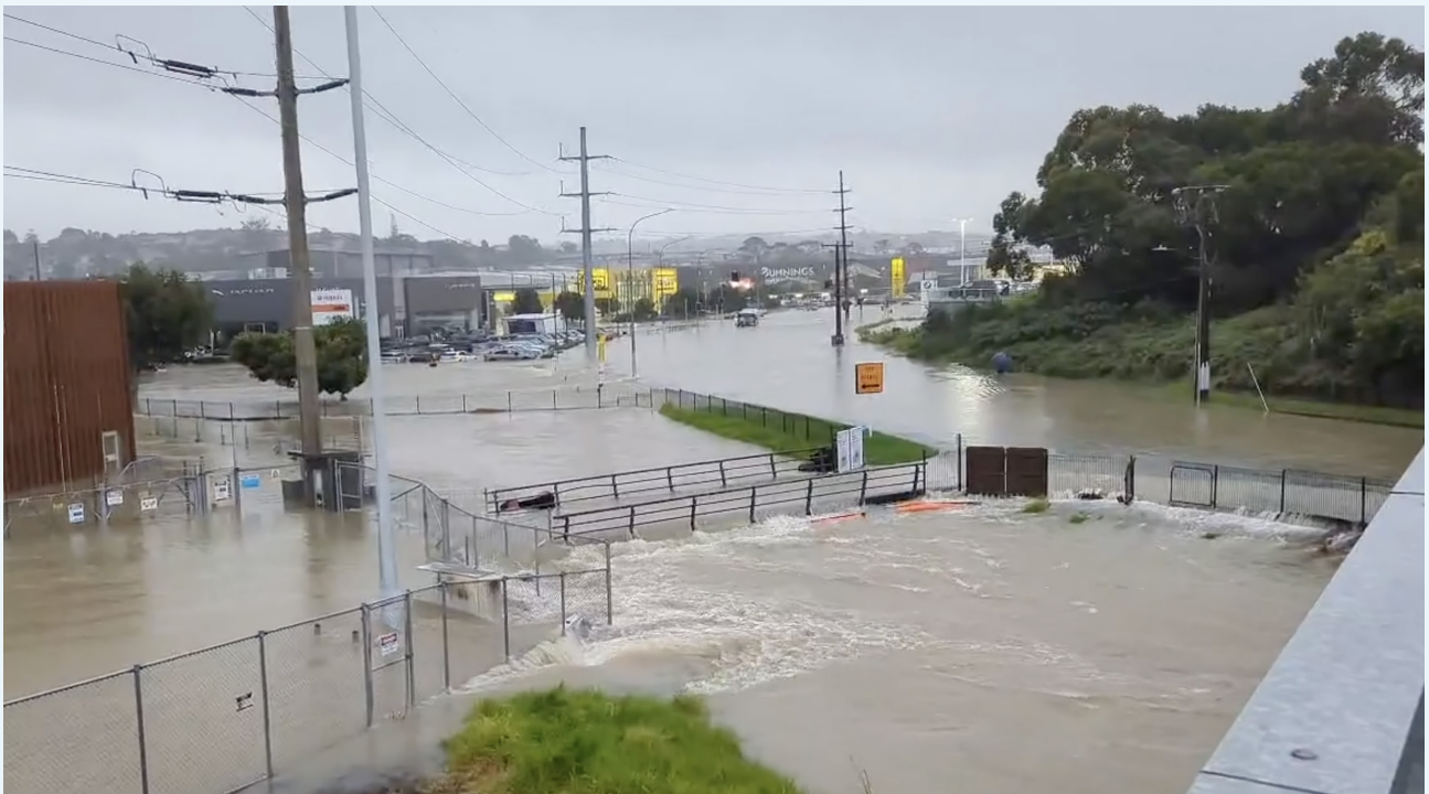
Wairau Pump Station, Auckland Anniversary floods 2023
