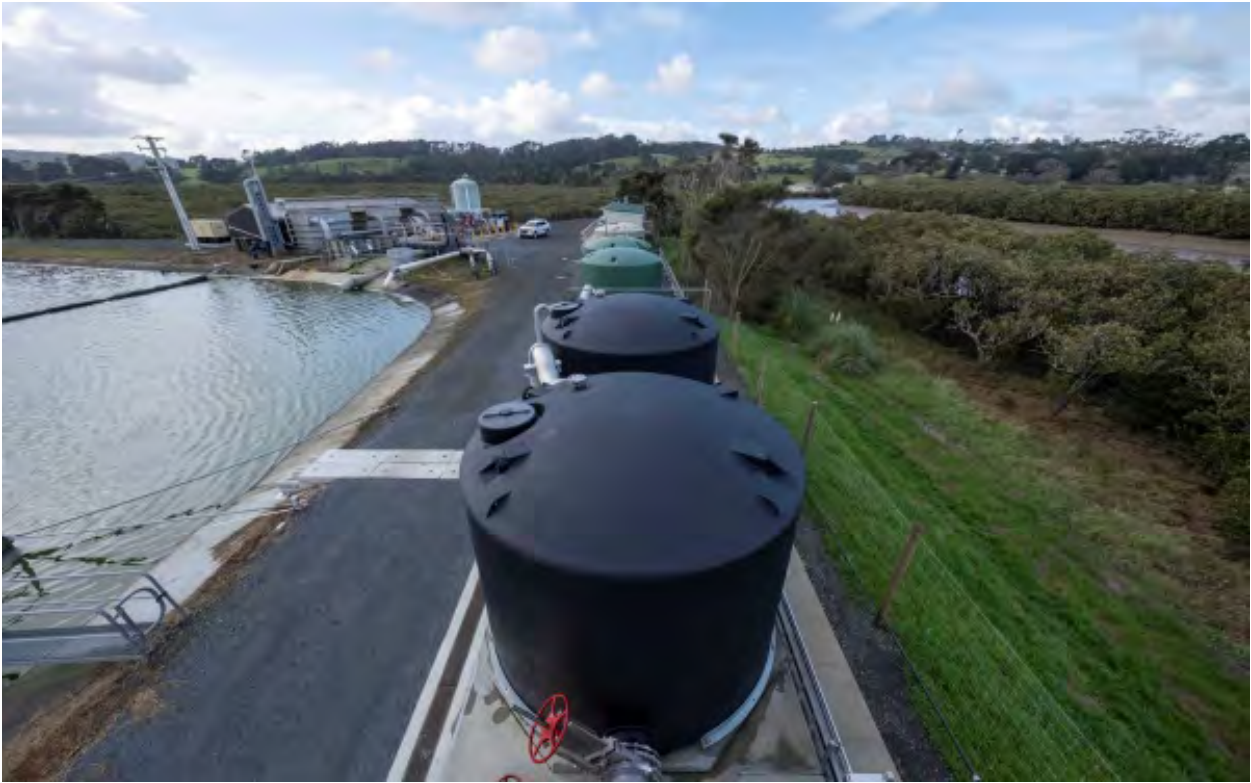
Figure 19 - Membrane aerated biofilm reactor (MABR) at Te Awaroa (Helensville)'s wastewater treatment plant
