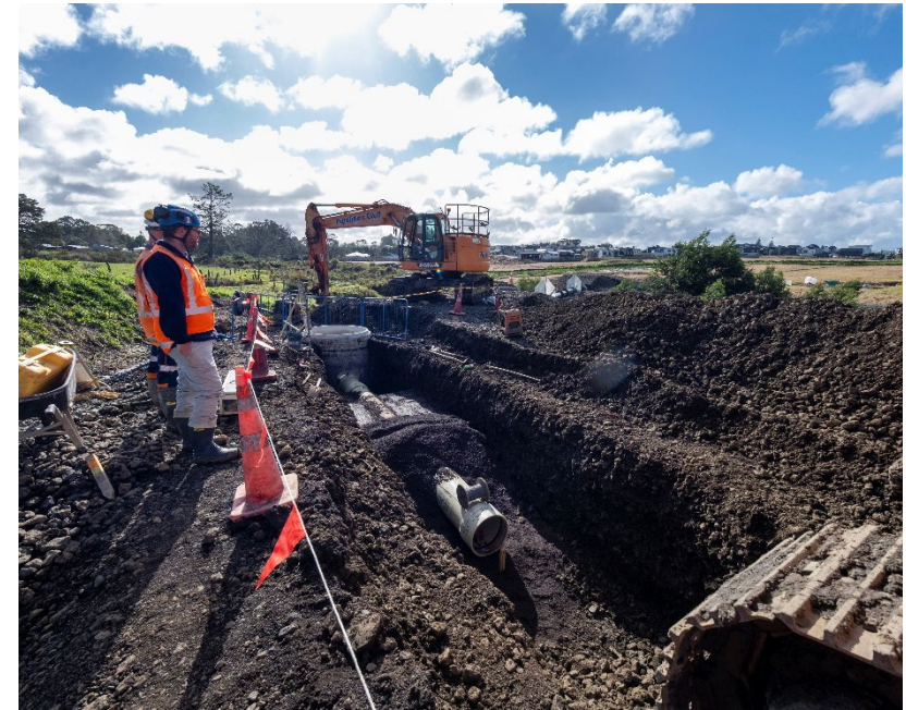
Northern Interceptor one - it's the new wastewater pipe that will connect Redhills to our network
