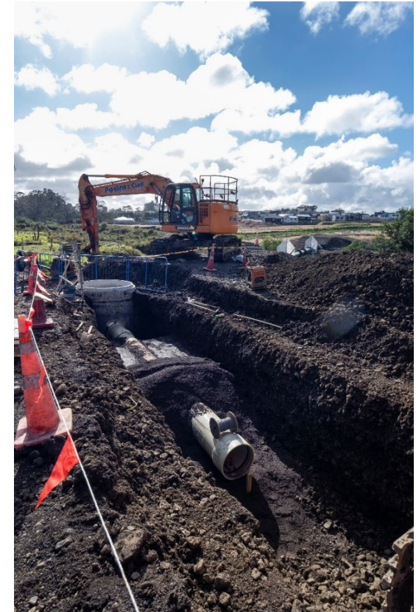
The new Northern Interceptor wastewater pipe that will connect Redhills to our network
