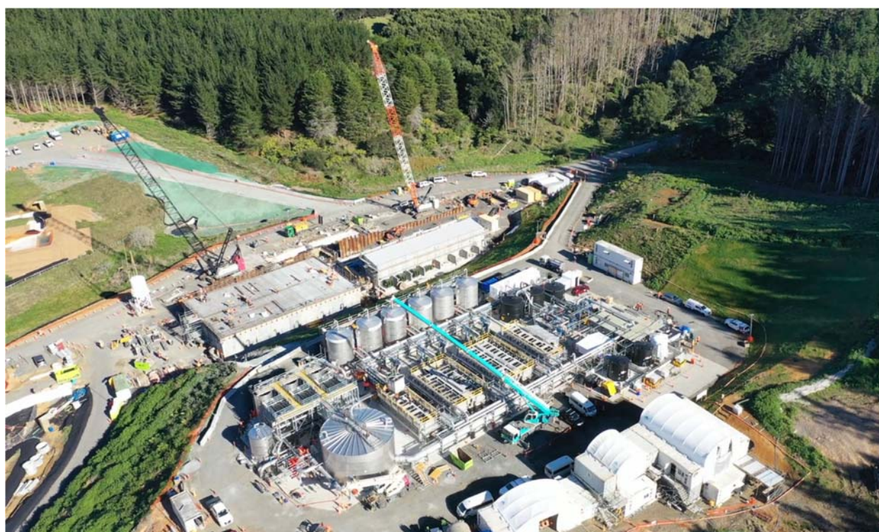
Our newly completed Waikato 50 water treatment plant
